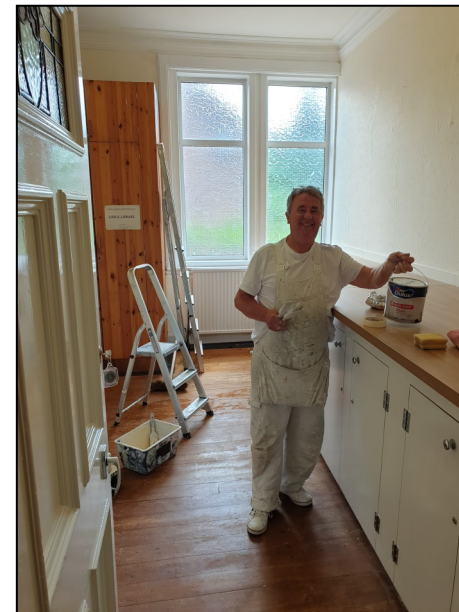
Norrie Telfer completing the internal work.
